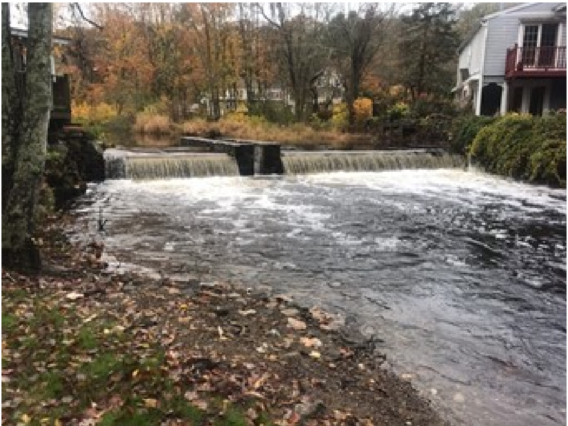
5-11. The completed Dolan Pond Fishway on the Falls River in Centerbrook Village, Essex, CT.
